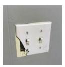
Some fittings are cracked or damaged
