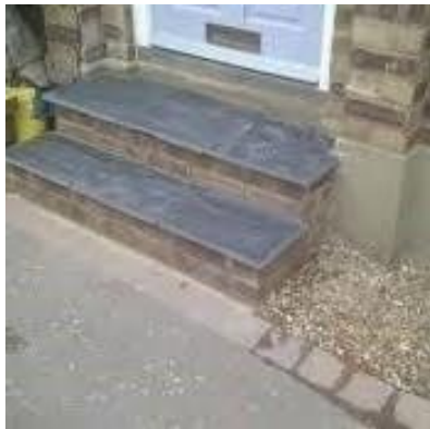
Steps up to external doors
